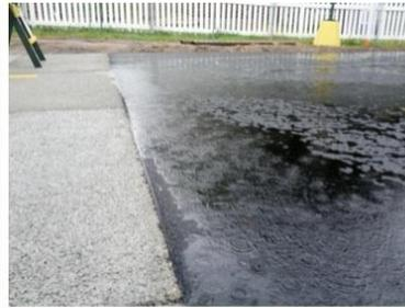
*Visible difference between the traditional asphalt pavement and pervious concrete pavement during rains*
