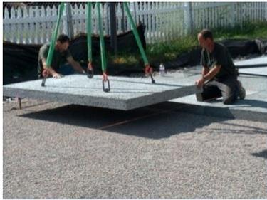
*Removable pervious concrete slab is being installed*
