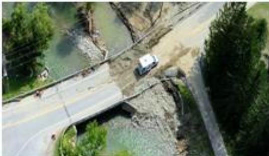
*Image left:* Bridge damage in southern Vermont as a result of flooding incurred during Hurricane Irene. Image source: Mansfield Flight LLC.
